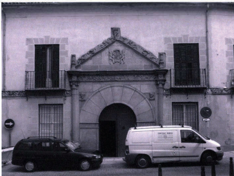
Figure 21. Façade of the Palace of Valdeaguila
